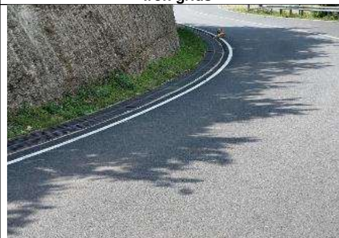
Figure 9. Covered drainage channels with an iron grids
